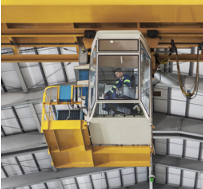
2,100 cameras to oversee a safe operating environment. The assessment of worker distance from suspended loads is one of the functionalities comprising an early alarm system.
