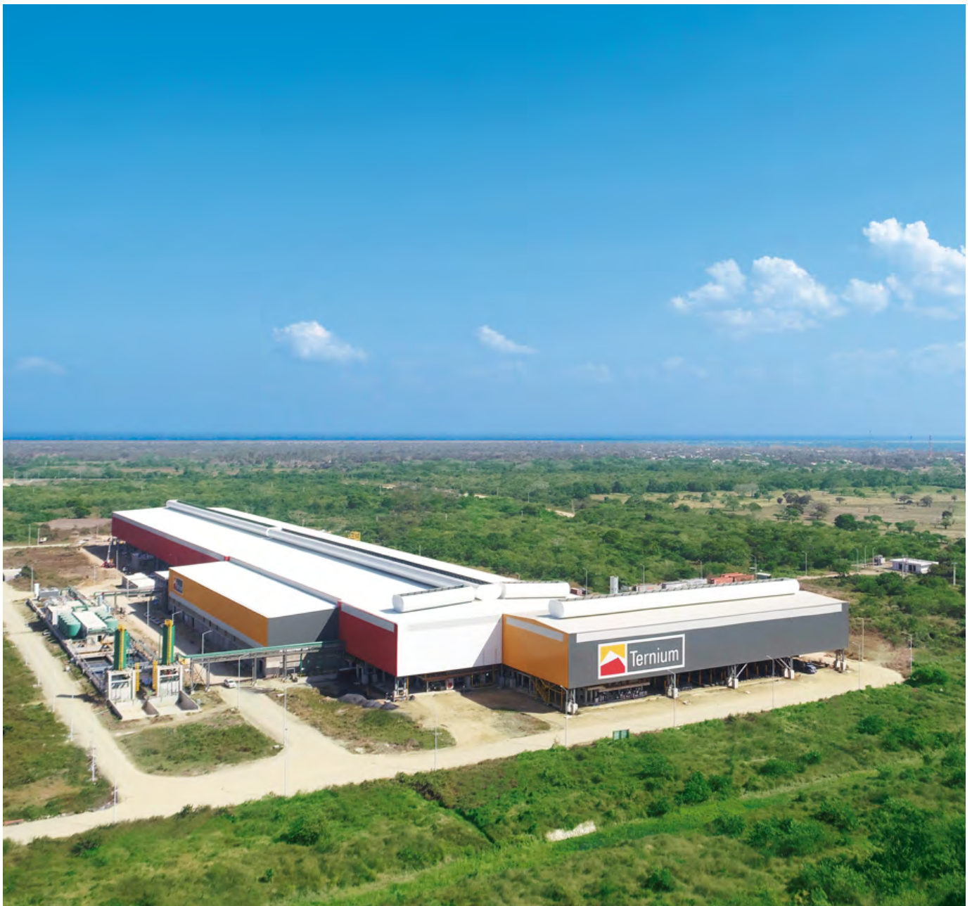
New facility at Palmar de Varela, Colombia. The 520,000 tons-per-year capacity mill has incorporated three shifts since its start-up in November 2020.
